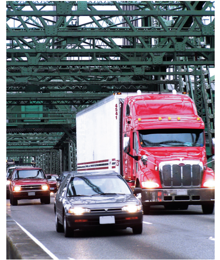
Cars and trucks move north on I-5 across the Columbia River. This project will improve travel efficiency for both commuters and freight haulers.
