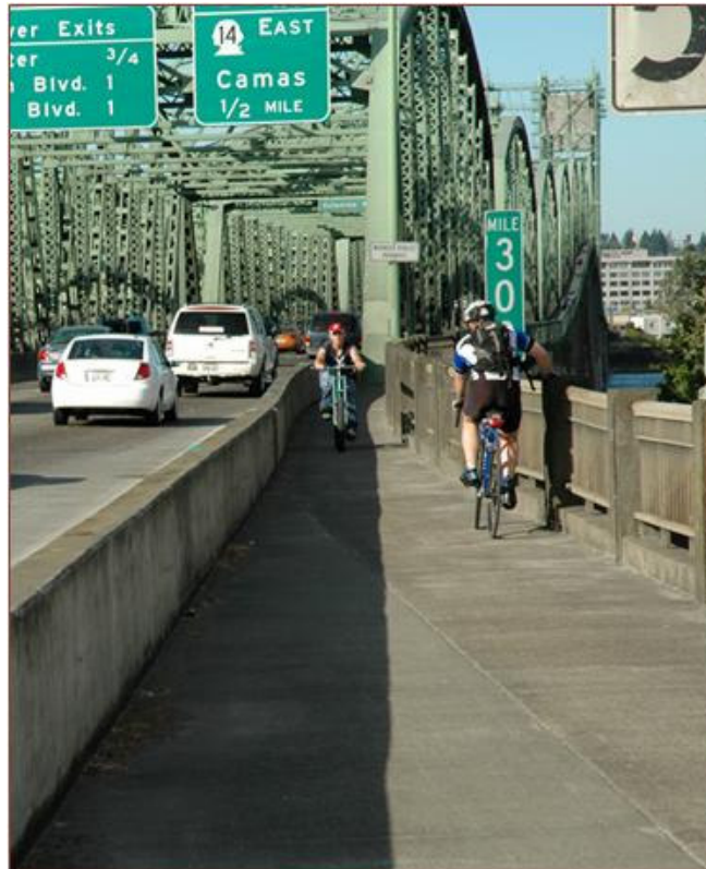
Figure 3-17. Photograph of Existing Non-Standard Multi-Use Pathway
