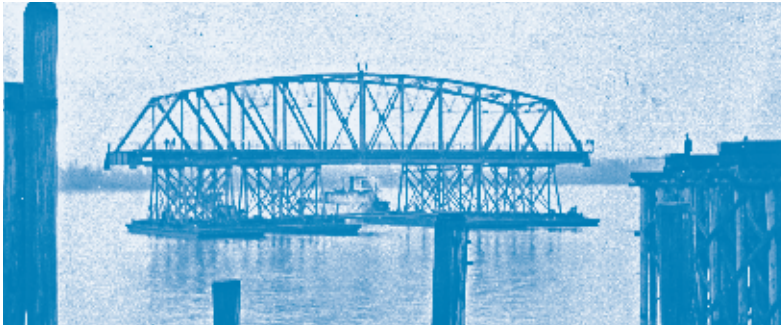
Bridge span is floated into place by barge during construction of the 1917 Interstate Bridge Oregon Historical Society, OrHi 101203
