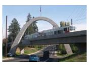
The City of Hillsboro did not want a pier in the center of the street, so a light rail bridge was built with a dramatic overhead arch straddling the road and the track.
